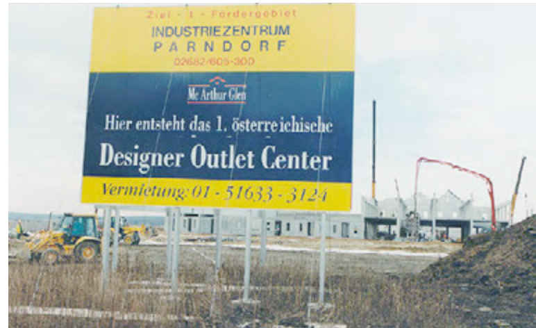
Baubeginn Designer Outlet Parndorf.
